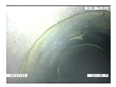
Code: Description: Broken Distance (ft): 8.6 Structural Grade: 4 0 O&M Grade: Clock Start/From: 12 Clock To: 12 1st Value: 2nd Value: Value Percent: Continuous Index: F01 Within 8" of Joint: YES
