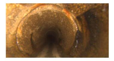
Code: CL Description: **Crack Longitudinal** Distance (ft): 27.9 Structural Grade: 2 O&M Grade: 0 Clock Start/From: 3 Clock To: 1st Value: 2nd Value: Value Percent: Continuous Index:
