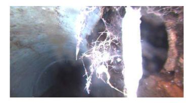
Code: TBD Description: **Tap Break-in Defective** Distance (ft): 31.2 Structural Grade: 0 O&M Grade: 3 Clock Start/From: 3 Clock To: 1st Value: 4.000 2nd Value: Value Percent: Continuous Index:
