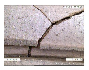
В Code: Description: Broken Distance (ft): 5.8 Structural Grade: 4 O&M Grade: 0 Clock Start/From: 11 3 Clock To: 1st Value: 2nd Value: Value Percent: Continuous Index: Within 8" of Joint: YES
