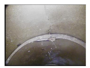
Code: CL Description: **Crack Longitudinal**
