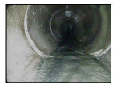
Code: MSA Description: Abandoned Survey Distance (ft): 127.4 Structural Grade: 0 O&M Grade: 0 Clock Start/From: Clock To: 1st Value: 2nd Value: Value Percent: Continuous Index: Within 8" of Joint: NO Remarks: encrustation
