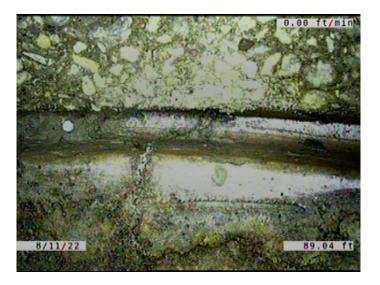
Code: MMC Description: **Miscellaneous Material Change** 89.0 Distance (ft): Structural Grade: 0 O&M Grade: 0 Clock Start/From: Clock To: 1st Value: 2nd Value: Value Percent: Continuous Index: Within 8" of Joint: NO Remarks: CONCRETE TO VCP
