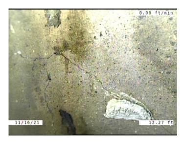
Code: CM Description: **Crack Multiple** Distance (ft): 12.3 Structural Grade: 3 O&M Grade: 0 Clock Start/From: 2 Clock To: 10 1st Value: 2nd Value: Value Percent: Continuous Index: Within 8" of Joint: YES
