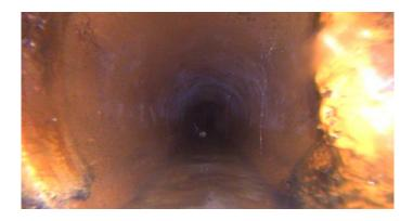
Code:DAZDescription:Deposits Attached OtherDistance (ft):41.3Structural Grade:0O&M Grade:2Clock Start/From:7Clock To:51st Value:1
