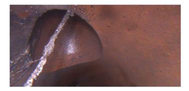
Code: TFD Description: Tap Factory Defective Distance (ft): 13.7 Structural Grade: 0
