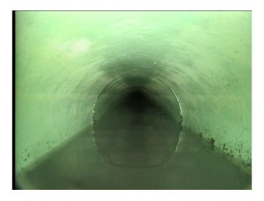
Code: MSA Description: Abandoned Survey Distance (ft): 188.7 Structural Grade: 0 O&M Grade: 0 Clock Start/From: Clock To: 1st Value: 2nd Value: Value Percent: Continuous Index: Within 8" of Joint: NO Remarks: **Heavy sediment**
