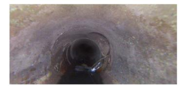
Code: MMC Description: **Material Change** Distance (ft): 134.8 Structural Grade: 0 O&M Grade: 0 Clock Start/From: Clock To: 1st Value: 2nd Value: Value Percent: Continuous Index: Within 8" of Joint: NO Remarks: pvc
