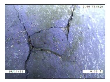
Code: Description: Broken Distance (ft): .3 Structural Grade: 4 O&M Grade: 0 Clock Start/From: 8 Clock To: 4 1st Value: 2nd Value: Value Percent: Continuous Index: Within 8" of Joint: YES
