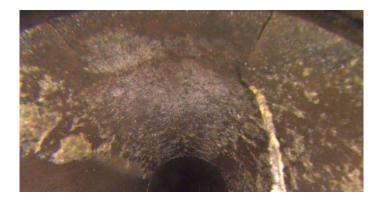
Code:CLDescription:Crack LongitudinalDistance (ft):9.3Structural Grade:2O&M Grade:0Clock Start/From:1
