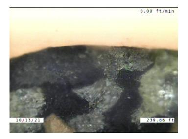
Code: Description: RPPD Point Repair Patch Patch Defective
