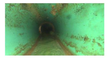
Code: MWL Description: Water Level Distance (ft): .0 Structural Grade: 0 O&M Grade: 0 Clock Start/From: Clock To: 1st Value: 2nd Value: Value Percent: 10.000 Continuous Index: Within 8" of Joint: NO
