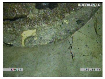
Code: MGO Description: **Miscellaneous General Observation** Distance (ft): 193.4 Structural Grade: 0 0 O&M Grade: Clock Start/From: Clock To: 1st Value: 2nd Value: Value Percent: Continuous Index: Within 8" of Joint: NO Remarks: MANHOLE FRAME HAS SHIFTED. SOIL VISIBLE.
