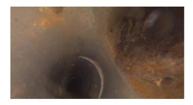
Code: TFD **Tap Factory Defective** Description: 52.6 Distance (ft): Structural Grade: 0 O&M Grade: 2 Clock Start/From: 2 Clock To: 1st Value: 4.000 2nd Value: Value Percent: Continuous Index: Within 8" of Joint:
