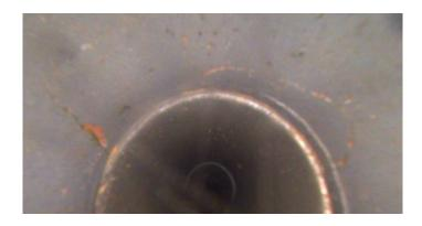
Code: CM Description: Crack Multiple Distance (ft): 61.3 Structural Grade: 3 O&M Grade: 0
