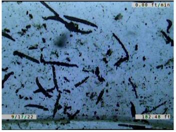
Code: MGO Description: **Miscellaneous General Observation** Distance (ft): 182.5 Structural Grade: 0 O&M Grade: 0 Clock Start/From: Clock To: 1st Value: 2nd Value: Value Percent: Continuous Index: Within 8" of Joint: NO JOINT/ PIPES NOT PUSHED ALL THE Remarks: WAY TOGETHER WHEN INSTALLED
