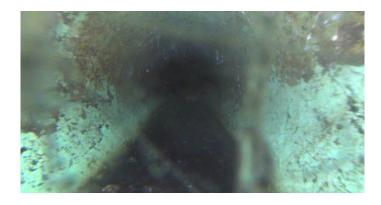
Code: MMC Description: **Material Change** Distance (ft): 159.8 Structural Grade: 0 O&M Grade: 0 Clock Start/From: Clock To: 1st Value: 2nd Value: Value Percent: Continuous Index: Within 8" of Joint: NO Remarks: PVC
