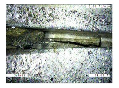
Code: IDJ Description: **Infiltration Dripper Joint** Distance (ft): 34.6 Structural Grade: 0 O&M Grade: 3 Clock Start/From: 3 Clock To: 1st Value: 2nd Value: Value Percent: Continuous Index: Within 8" of Joint: YES Remarks:
