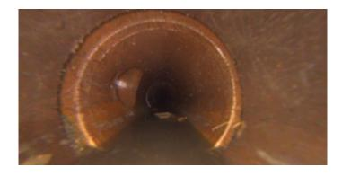
Code:RFBDescription:Roots Fine BarrelDistance (ft):32.5Structural Grade:0O&M Grade:2Clock Start/From:4Clock To:11st Value:1
