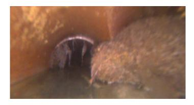
Code: TFD **Tap Factory Defective** Description: Distance (ft): 83.0 Structural Grade: 0 O&M Grade: 2 Clock Start/From: 3 Clock To: 1st Value: 4.000 2nd Value: Value Percent: Continuous Index:
