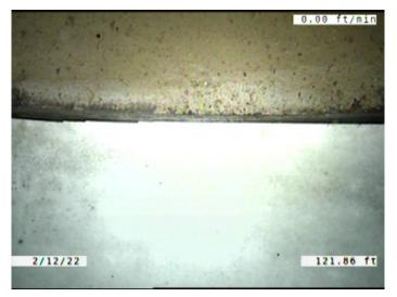
Code: MMC Description: **Miscellaneous Material Change** Distance (ft): 121.9 Structural Grade: 0 O&M Grade: 0 Clock Start/From: Clock To: 1st Value: 2nd Value: Value Percent: Continuous Index: Within 8" of Joint: NO Remarks: VCP TO PVC
