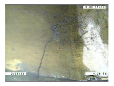
Code: CM Description: **Crack Multiple** Distance (ft): 4.3 Structural Grade: 3 O&M Grade: 0 Clock Start/From: 12 Clock To: 12 1st Value: 2nd Value: Value Percent: Continuous Index: **S01** Within 8" of Joint: YES
