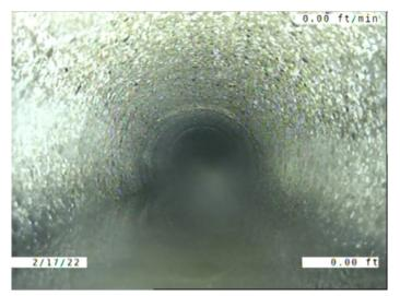
Code: SAV Description: **Surface Damage Aggregate Visible** Distance (ft): .0 Structural Grade: 2 O&M Grade: 0 Clock Start/From: 8 Clock To: 4 1st Value: 2nd Value: Value Percent: **S06** Continuous Index:
