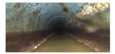
Code:LFWDescription:Lining Failure Wrinkled
