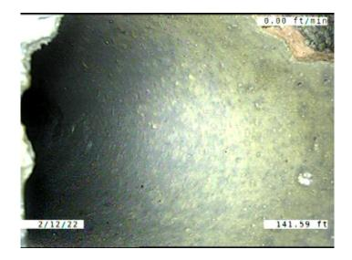
Code: TBD Description: Tap Break-in/Hammer Defective Distance (ft): 141.6 Structural Grade: 0 O&M Grade: 3 Clock Start/From: 10 Clock To: 1st Value: 6.000 2nd Value: Value Percent: Continuous Index: Within 8" of Joint: NO Remarks: HSV in Tap
