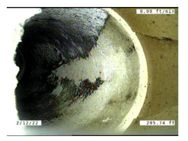
Code: TBD Description: Tap Break-in/Hammer Defective Distance (ft): 205.7 Structural Grade: 0 O&M Grade: 3 Clock Start/From: 10 Clock To: 1st Value: 6.000 2nd Value: Value Percent: Continuous Index: Within 8" of Joint: NO Remarks: HSV in tap
