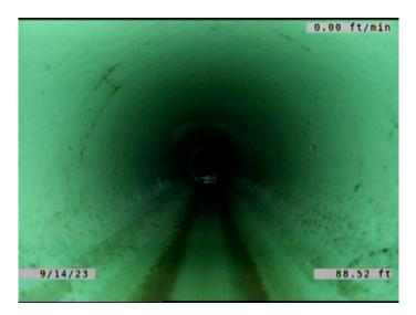
Code: MWLS Description: **Miscellaneous Water Level Sag** Distance (ft): 88.5 Structural Grade: 2 O&M Grade: 0 Clock Start/From: Clock To: 1st Value: 2nd Value: 5.000 Value Percent: Continuous Index: F03 Within 8" of Joint: NO
