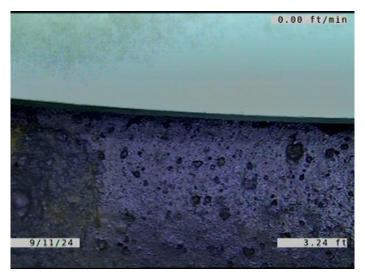
Code: JOMD Description: Joint Offset Medium Defective 3.2 Distance (ft): Structural Grade: 3 O&M Grade: 0 Clock Start/From: Clock To: 1st Value: 2nd Value: Value Percent: Continuous Index: Within 8" of Joint: NO Remarks:
