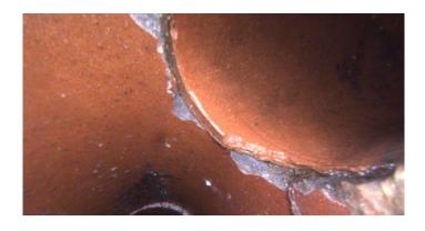
Code: TBD Description: **Tap Break-in Defective** Distance (ft): 22.5 Structural Grade: 0 O&M Grade: 3 Clock Start/From: 2 Clock To: 1st Value: 4.000 2nd Value: Value Percent: Continuous Index:
