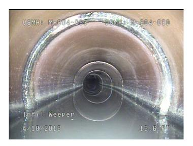
Code: IW Description: Infil Weeper Distance (ft): 13.6 Structural Grade: 0 O&M Grade: 2 Clock Start/From: 12 Clock To: 12 1st Value: 2nd Value: Value Percent: Continuous Index: **S01** Within 8" of Joint: YES
