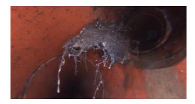
Code: TFD Description: **Tap Factory Defective** Distance (ft): 68.9 Structural Grade: 0 O&M Grade: 2 Clock Start/From: 10 Clock To: 1st Value: 4.000 2nd Value: Value Percent: Continuous Index: Within 8" of Joint:
