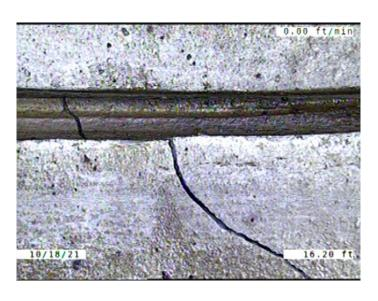
В Code: Description: Broken Distance (ft): 16.2 Structural Grade: 4 O&M Grade: 0 Clock Start/From: 2 3 Clock To: 1st Value: 2nd Value: Value Percent: Continuous Index: Within 8" of Joint: YES
