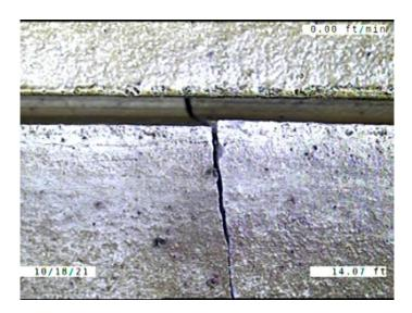
Code: Description: Broken Distance (ft): 14.1 Structural Grade: 4 O&M Grade: 0 Clock Start/From: 2 Clock To: 4 1st Value: 2nd Value: Value Percent: Continuous Index: Within 8" of Joint: YES Remarks:
