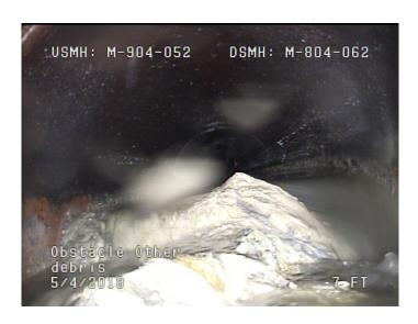
Code: OBZ Description: **Obstacle Other** 7.0 Distance (ft): Structural Grade: 0 O&M Grade: 5 Clock Start/From: 3 Clock To: 8 1st Value: 2nd Value: Value Percent: 45.000 Continuous Index: Within 8" of Joint: NO Remarks: debris
