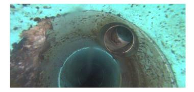
Code:DAGSDescription:Deposits Attached GreaseDistance (ft):53.8Structural Grade:0O&M Grade:2Clock Start/From:10Clock To:111st Value:22nd Value:1
