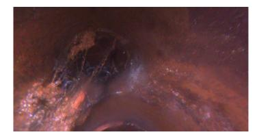
Code: TFD **Tap Factory Defective** Description: Distance (ft): 102.2 Structural Grade: 0 O&M Grade: 2 Clock Start/From: 1 Clock To: 1st Value: 4.000 2nd Value: Value Percent: Continuous Index: Within 8" of Joint:
