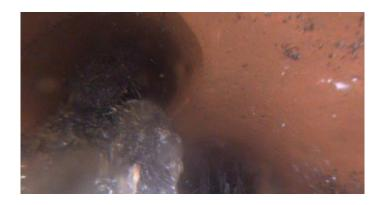
Code: TFD Description: **Tap Factory Defective** Distance (ft): 154.0 Structural Grade: 0 O&M Grade: 2 Clock Start/From: 10 Clock To: 1st Value: 4.000 2nd Value:
