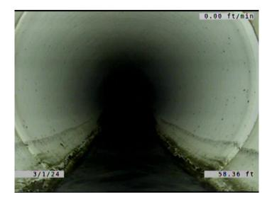
Code: MWLS Description: **Miscellaneous Water Level Sag** Distance (ft): 58.4 Structural Grade: 2 O&M Grade: 0 Clock Start/From: Clock To: 1st Value: 2nd Value: 15.000 Value Percent: Continuous Index: F01 Within 8" of Joint: NO
