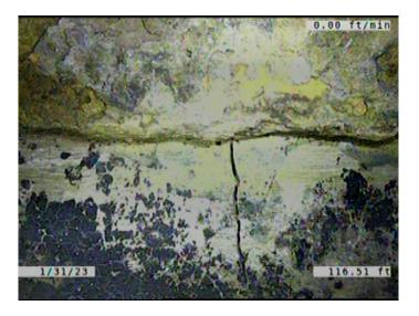
Code: MMC Description: **Miscellaneous Material Change** Distance (ft): 116.5 Structural Grade: 0 O&M Grade: 0 Clock Start/From: Clock To: 1st Value: 2nd Value: Value Percent: Continuous Index: Within 8" of Joint: NO DIP TO VCP Remarks:
