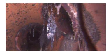
Code:TBDDescription:Tap Break-in DefectiveDistance (ft):2.8Structural Grade:0O&M Grade:3Clock Start/From:2Clock To:11st Value:4.000
