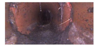
Code: DSF Description: **Deposits Settled Fine** Distance (ft): .0 Structural Grade: 0 2 O&M Grade: Clock Start/From: 6 Clock To: 1st Value: 2nd Value: 5.000 Value Percent:
