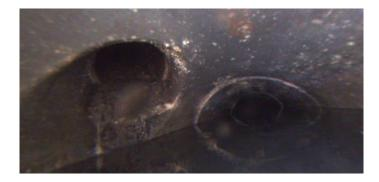
Code: TFD Description: **Tap Factory Defective** Distance (ft): 252.7 Structural Grade: 0 O&M Grade: 2 Clock Start/From: 2 Clock To: 1st Value: 4.000 2nd Value: Value Percent: Continuous Index:
