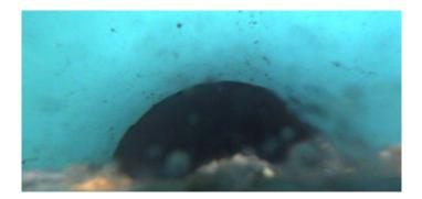
Code: MMC Description: **Material Change** Distance (ft): 2.7 Structural Grade: 0 O&M Grade: 0 Clock Start/From: Clock To: 1st Value: 2nd Value: Value Percent: Continuous Index: Within 8" of Joint: NO
