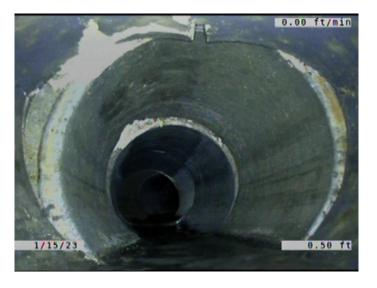
Code: DR Description: **Deformed Rigid** Distance (ft): .5 Structural Grade: 5 O&M Grade: 0 Clock Start/From: Clock To: 1st Value: 2nd Value: 10.000 Value Percent: Continuous Index: Within 8" of Joint: NO Remarks:
