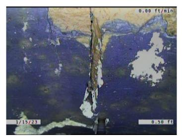
Code: Description: Broken Distance (ft): .5 Structural Grade: 4 0 O&M Grade: Clock Start/From: 12 Clock To: 12 1st Value: 2nd Value: Value Percent: Continuous Index:
