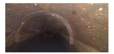
Distance (ft): 4.4 Structural Grade: 3 O&M Grade: 0 Clock Start/From: 9 Clock To: 3 1st Value: 2nd Value: Value Percent:
