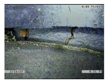
BVV Code: Description: **Broken Void Visible** Distance (ft): .3 Structural Grade: 5 0 O&M Grade: Clock Start/From: 12 Clock To: 12 1st Value: 2nd Value: Value Percent: Continuous Index: **S01**
