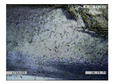
Code: JAL Description: Joint Angular Large 16.1 Distance (ft): Structural Grade: 4 O&M Grade: 0 Clock Start/From: Clock To: 1st Value: 2nd Value: Value Percent: Continuous Index: Within 8" of Joint: NO Remarks:
