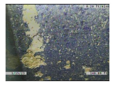
Code: SSS Description: Surface Damage Surface Spalling Distance (ft): 146.8 Structural Grade: 2 O&M Grade: 0 Clock Start/From: 9 Clock To: 1st Value: 2nd Value: Value Percent: Continuous Index: Within 8" of Joint: NO
