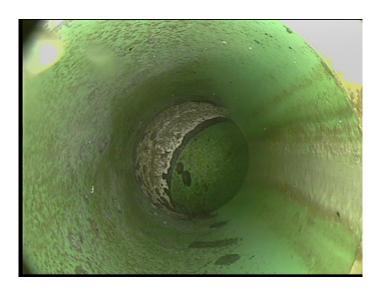
Code: TF Description: **Tap Factory** Distance (ft): 7.1 Structural Grade: 0 O&M Grade: 0 Clock Start/From: 2 Clock To: 1st Value: 4.000 2nd Value: Value Percent: Continuous Index: Within 8" of Joint: NO
