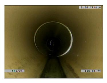
Code: MWLS Description: **Miscellaneous Water Level Sag** Distance (ft): 116.0 Structural Grade: 2 0 O&M Grade: Clock Start/From: Clock To: 1st Value: 2nd Value: Value Percent: 10.000 Continuous Index: F03 Within 8" of Joint: NO
